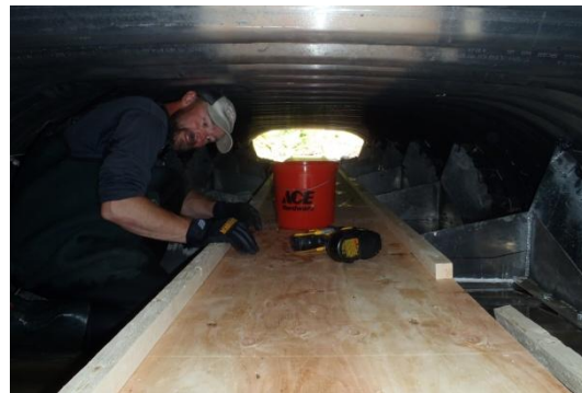
Tram system to fill culvert with rock
