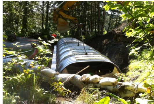
Tram system to fill culvert with rock
