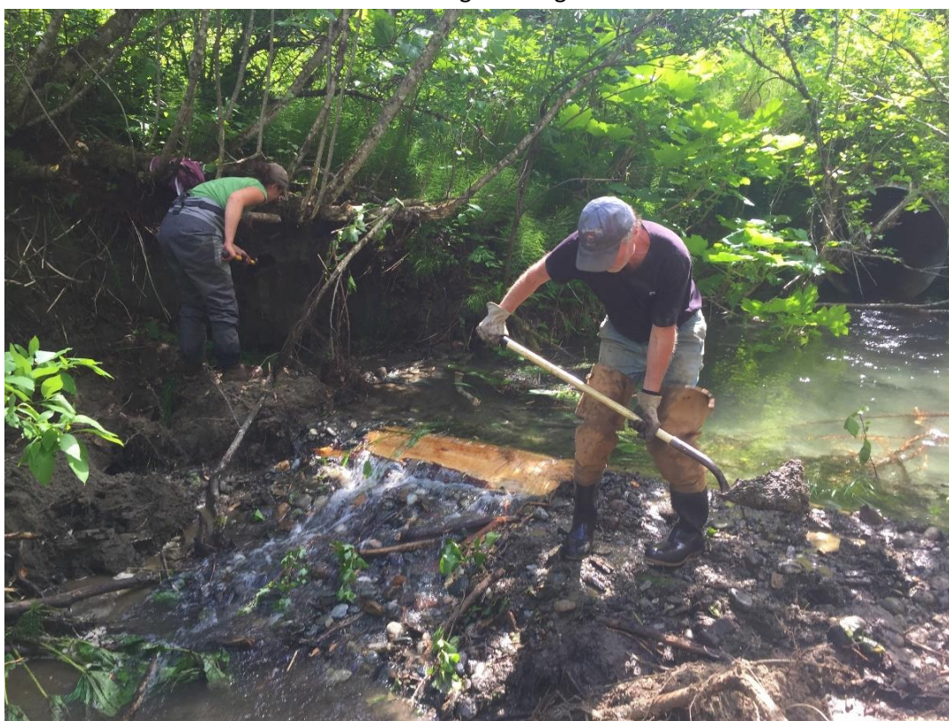
Shoring up weirs with hand tools.
