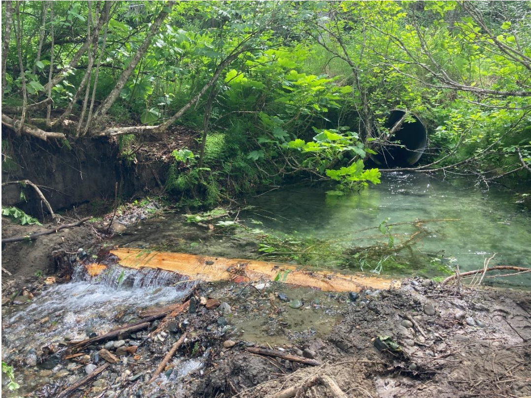
Resulting pool after first log is placed, embedded, and notched. Perch is resolved immediately!
