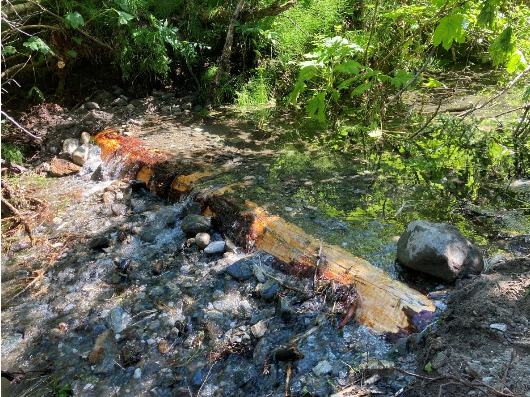
Resulting pool after second log is placed, embedded, and notched.
