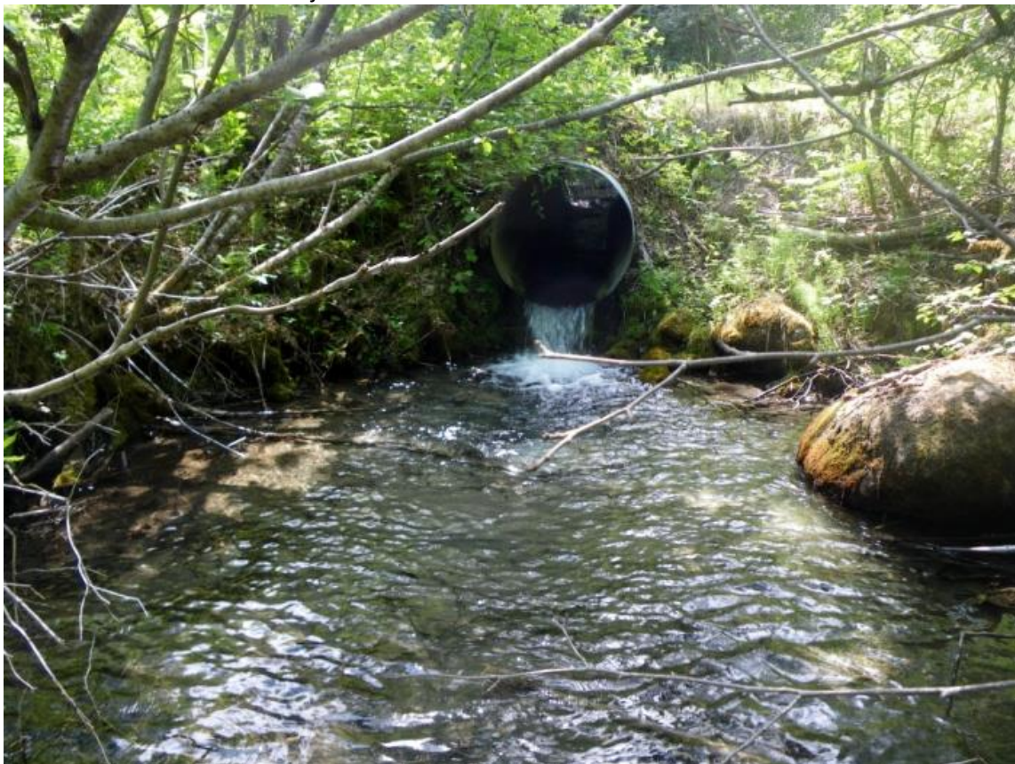
Pre-construction perch causing a barrier to fish passage.
