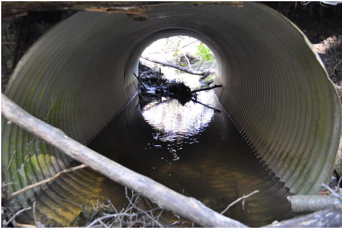
Woody debris collecting at culvert mouths, potentially impeding fish passage. 5/13/2020
