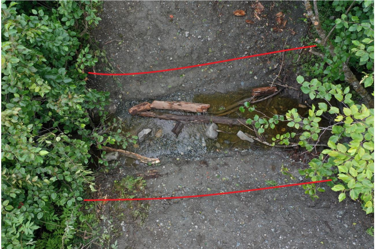
Newly-constructed channel showing designed bank-full limits (red lines)
